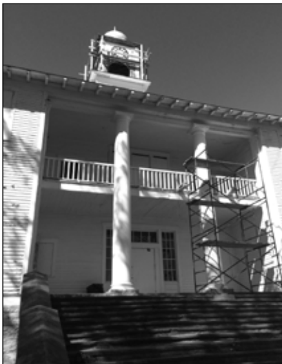
The rehabilitation of Lincoln Hall.
