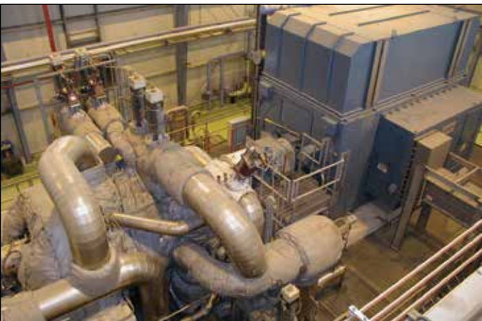
A boiler at Domtar in Hawesville that produces steam to generate electricity. Photo by Domtar
