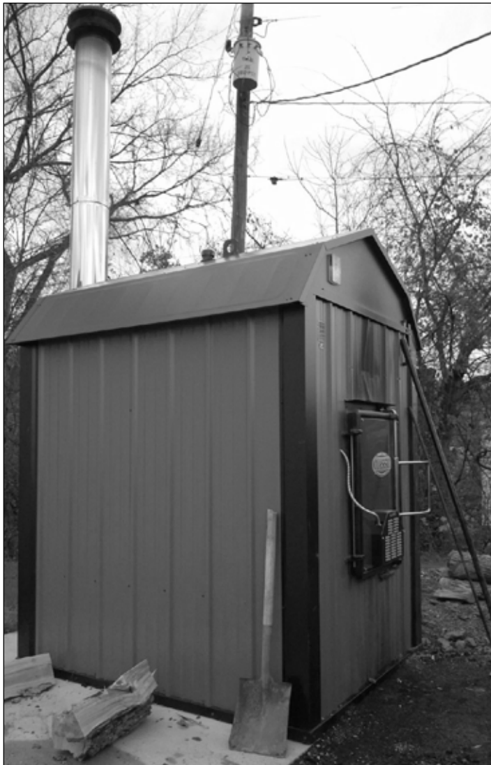
An outdoor wood boiler, or hydronic heater.
